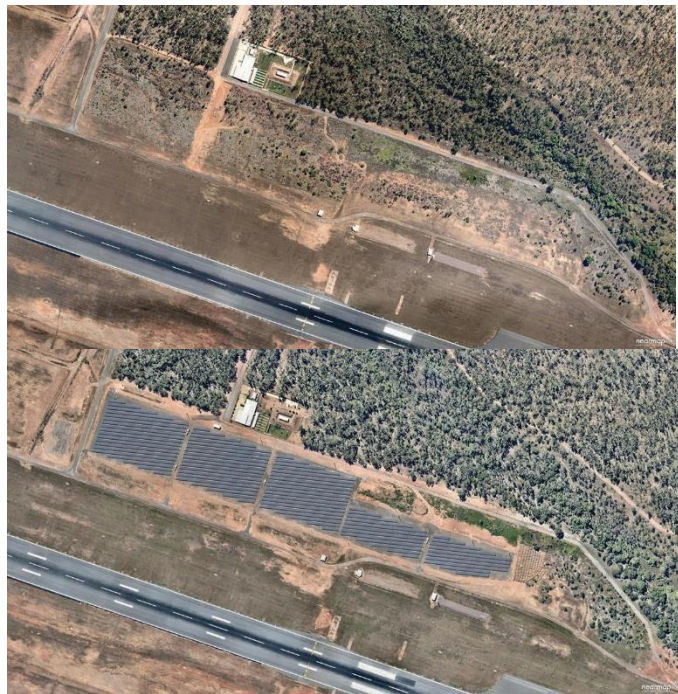
Darwin Airport Solar Project Stage 1, before and after
